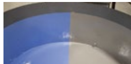
POTABLE WATER TANKS
