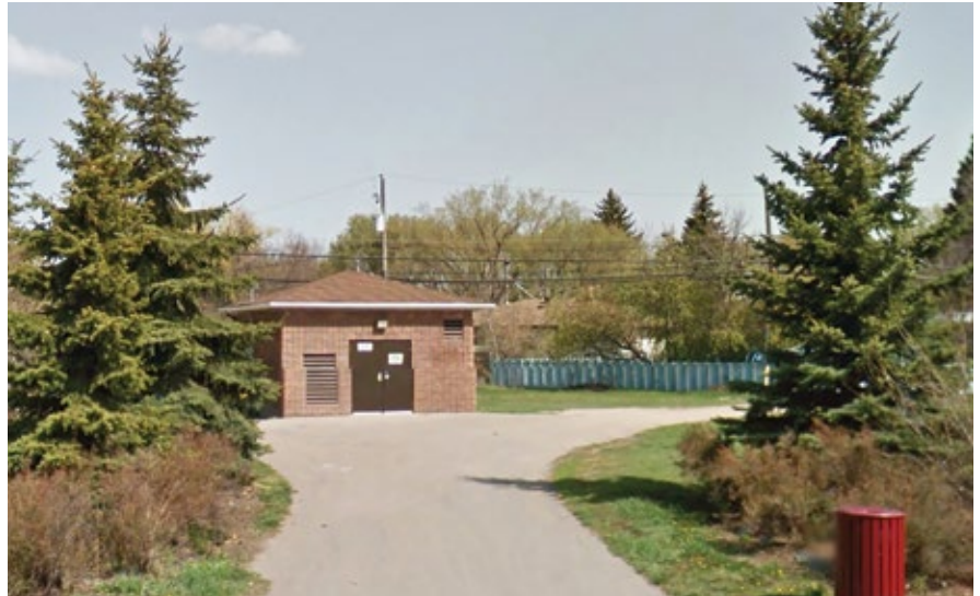
25th Avenue lift station
